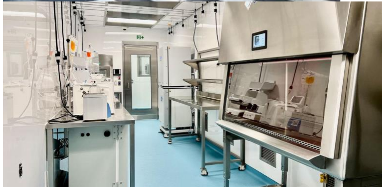
Figures 2& 3: GermFree mobile laboratories that are GMP-grade to produce CAR-T cell therapies. Source: https://www.germfree.com/facilities/mobile-cgmp-cleanrooms/
